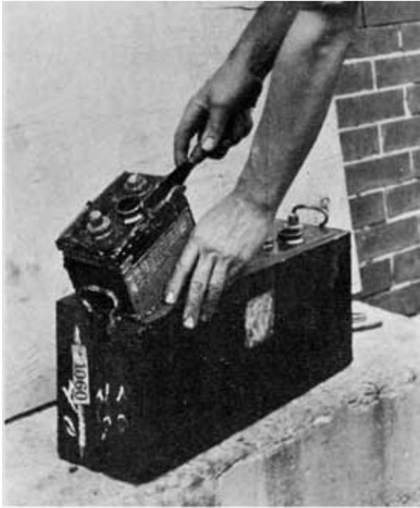
Fig. 198. Removing Compound from Cover
